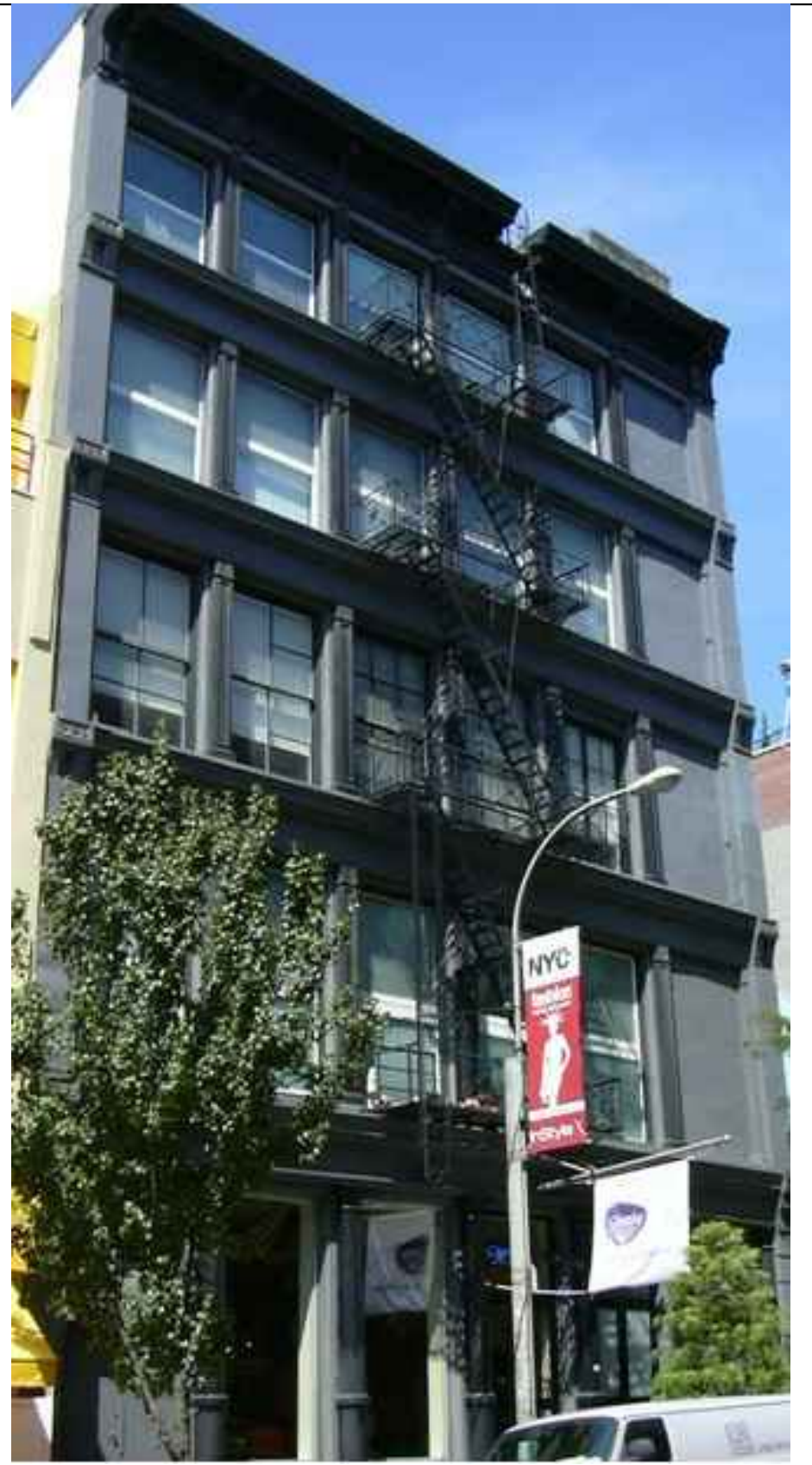
03 2010 LPC DESIGNATION PHOTO NTS
