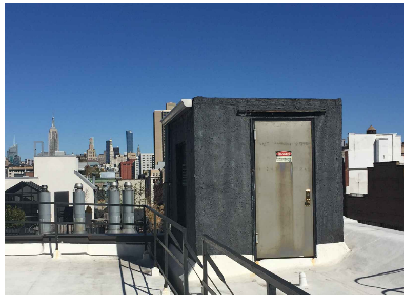
04 EXISTING BULKHEAD CONDITIONS NTS
