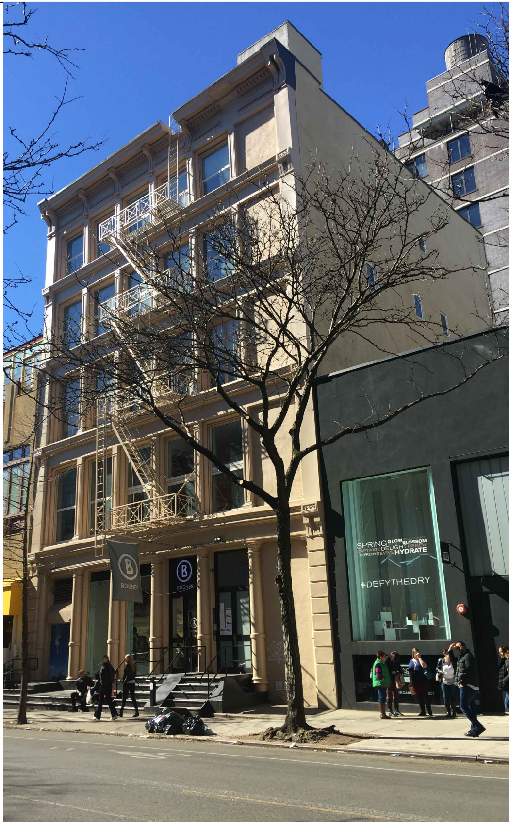
02 EXISTING VIEW FACING SOUTH NTS
